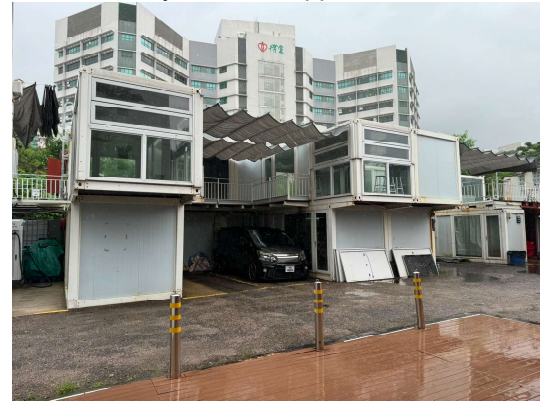
Photo 4: Block 2: Traffic Equipment Storage
